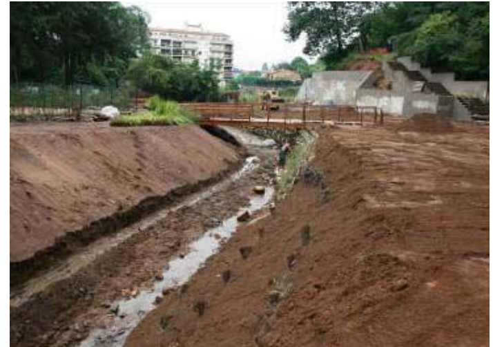
During the work
